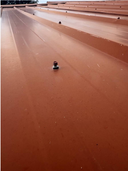
5 Screw in the pan. This is how this panel is fastened.
